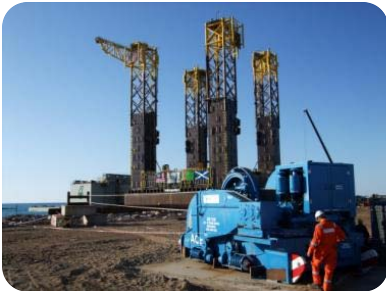
Load out of jacket and topsides offshore Turkmenistan in 2010 and 2011
